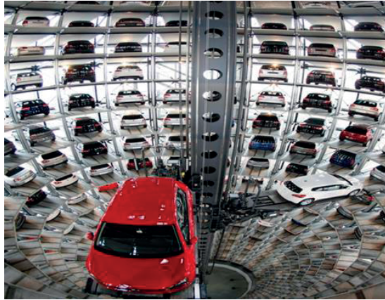
Fig. 3. High-tech CarTowers parking
