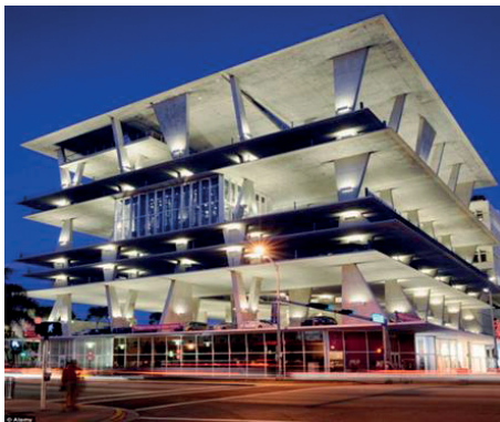
Fig. 2. The Miami – 1111 Lincoln Road parking lot
